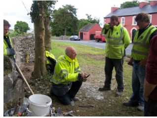
Traditional skills training in lime mortar and stonewall building
